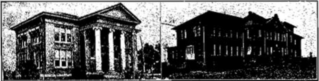
CARNEGIE LIBRARY, STATE A. & M. COLLEGE, TALLAHASSEE, FLA., MECHANICS ART BUILDING
