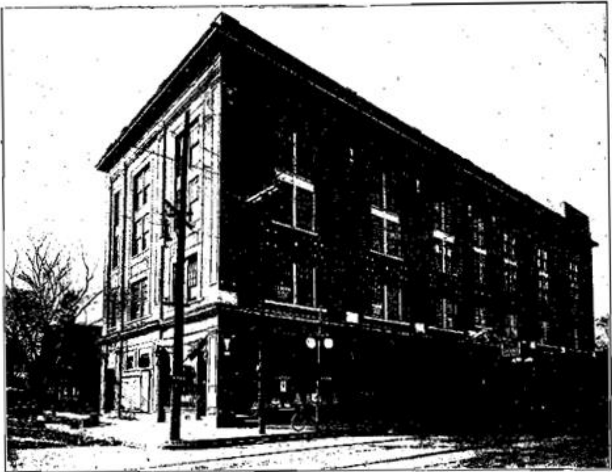
MOSAIC TEMPLARS' OFFICE BUILDING, LITTLE ROCK, ARKANSAS.
